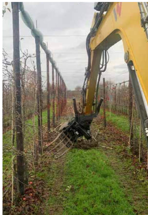
Picture 12. Steelwrist at work removing trees with structure in place under hail net system
