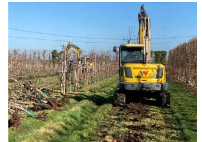
Picture 5. Orchard grubbing in progress at Wenderton Farm Ellis Contracting Services
